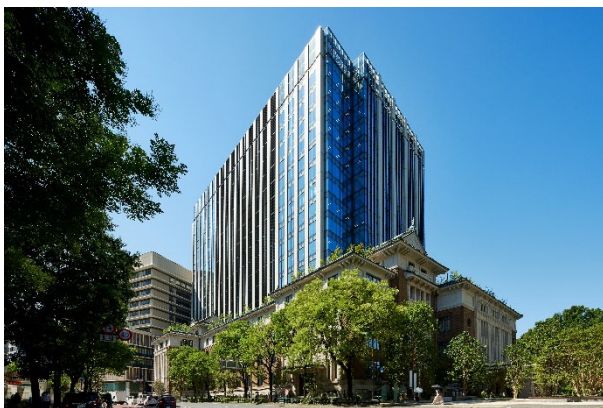
Exterior view of Kudan Kaikan Terrace
