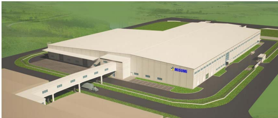
Illustration of Vietnam Plant No. 4 once completed
